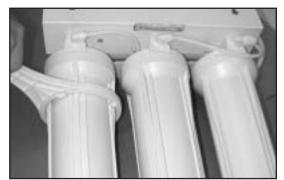
Figure 11 - Using sump wrench to change filter cartridges
