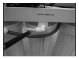
Figure 9 - Disconnect pre-carbon outlet tube from sump housing
