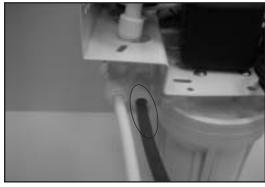
b. Connect the 3/8" blue tube from the **(90° elbow)** granular activated carbon post-filter fitting to the quick connect fitting on the threaded pipe on the spigot.
