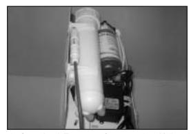
d. **Standard Faucet** - Connect the 1/4" red tube to the drain fitting.
