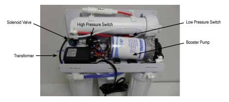
17. Locate the black and red wires coming from the pump. Follow these black and red wirers to the connector. On the other side of the connector cut the two black wires.
